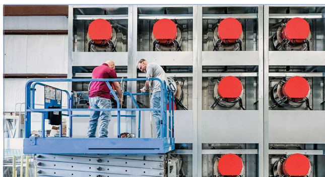
Motors used to power data center cooling equipment.
